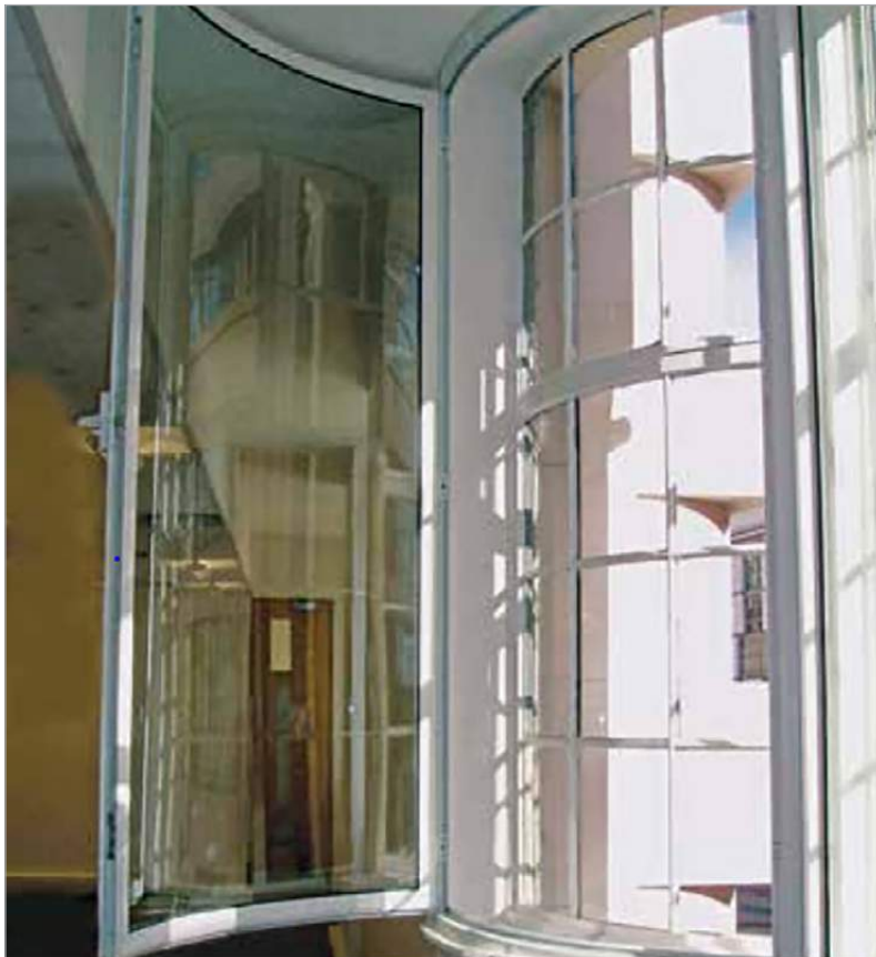
Secondary glazing can be made to fit unique windows so there is minimal harm to original features
