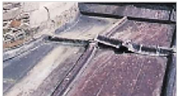
Splits in metal roofs or flashings should be repaired as soon as possible to prevent water ingress
