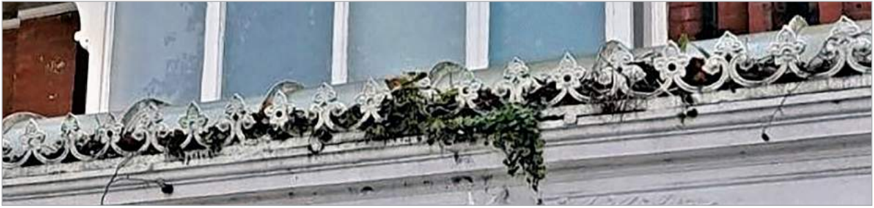
Blocked gutters cause water to overflow and can lead to issues with damp
