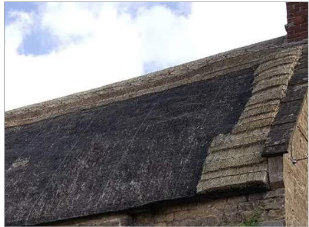
Patch repairs can be used to maintain thatch roofs
