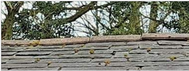
Cracked ridge tiles and missing mortar can lead to damp ingress
