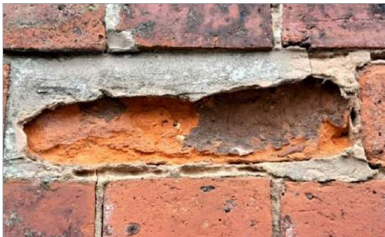
Using cement mortar can cause traditional bricks to corrode
