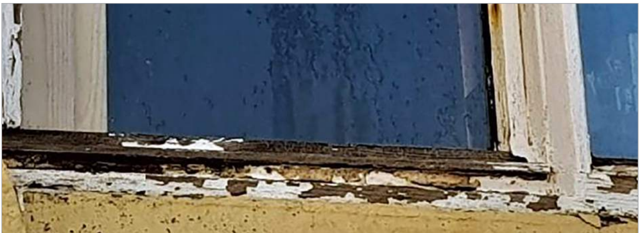
Timber windows should be repainted every 7 years to protect the wood from decaying
